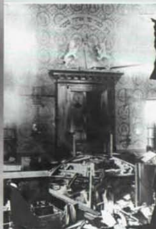
Destruction of synagogue in Eschwege, Germany (November 1938)
