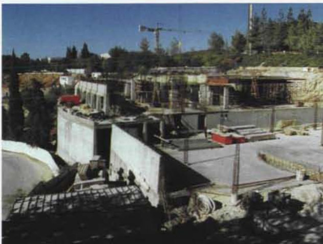
The Visitors Center, currently in the advanced stages of construction
